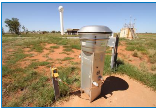
Figure 2-2: BoM Monitoring Station
