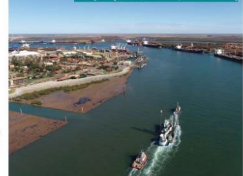
The dredge arriving at the Port of Port Hedland, prior to works commencing
