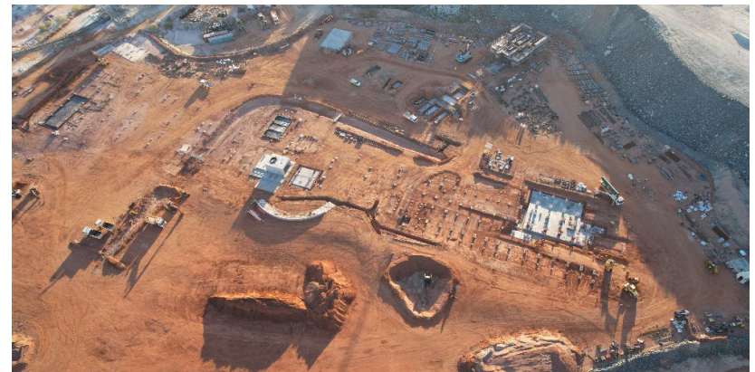
Crushing and ore sorting civil and concrete works July 2023
